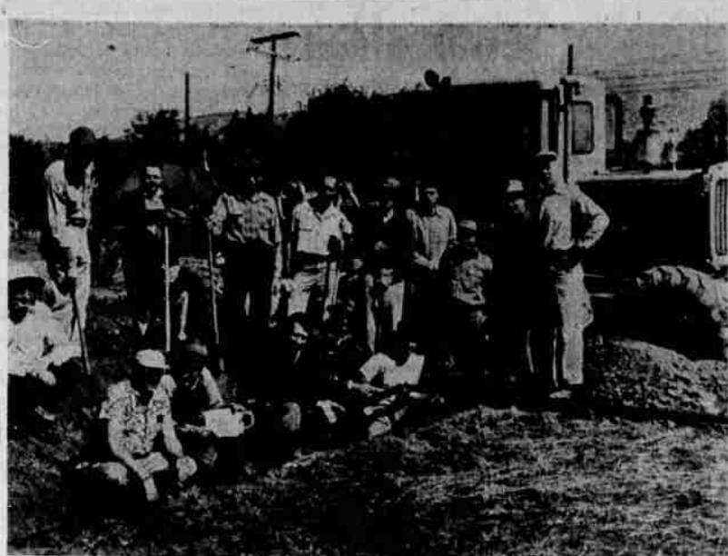
DIRT FLEW when this crew got busy on shovel handles for laying pipe at the new Kiwanis Park on Kit Carson Way last weekend. Hundreds of feet of pipe for the underground sprinkling system is being laid with volunteer help. This group was on hand Saturday. Front row, left to right, are Larry Brown, Mike Ladouceur, Local Union (plumbers) No. 191, Dick Pearson, Paul Hanna, plumber's union member, Floyd Wilson, resident manager of Carlson Products Corporation and Stan Miller, president of the Klamath Falls Kiwanis Club. Back row, same order, Dr. E. M. Causey, George Wardell, Vinc Bousquet, Marion Grant, Greer Drew, John Holzgang, John O'Neil and Lowell Kaup. "Red" Franklin is in the grader cab.
