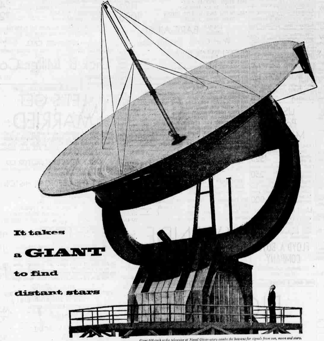
Giant 600-inch radio telescope at Naval Observatory combs the heavens for signals from sun, moon and stars.
