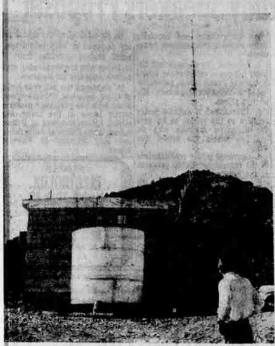
STATION MANAGER WALLY RICHARTZ looks over the newly completed transmitter room and antenna which is located atop a hill overlooking the OTI campus. The studio room is several hundred feet below the transmitter site. In front of the transmitter room is the large water storage tank which will be kept full for both domestic and fire protection purposes. Located at the 5,520-foot elevation, the top of the antenna extends 110 feet up from the mountain top. Transmission and co-axial cable connections can be seen extending from the transmitter room to the base of the antenna supports.
