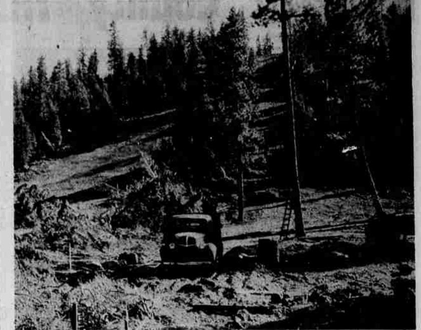
WORKMEN ARE NOW IN THE PROCESS of installing the power units and intermediate supports for the Poma-lift being installed at pictured new Tomahawk ski run. In addition to the steeply inclined run above, the new winter sports plant will include novice runs, ridge runs, and facilities for sledding. The trees pictured between the two clearings of the run will be removed, providing a 400-foot wide run at the lower elevations. The new sports area is located about 22 miles from Klamath Falls on the Lake of the Woods Highway.
