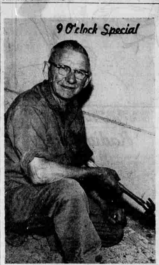
CHARLES FROST, 422 High Street, a maintenance man at Klamath Valley Hospital, was working on the building this morning and stopped for a break while the 9 o'clock photographer recorded the event.
