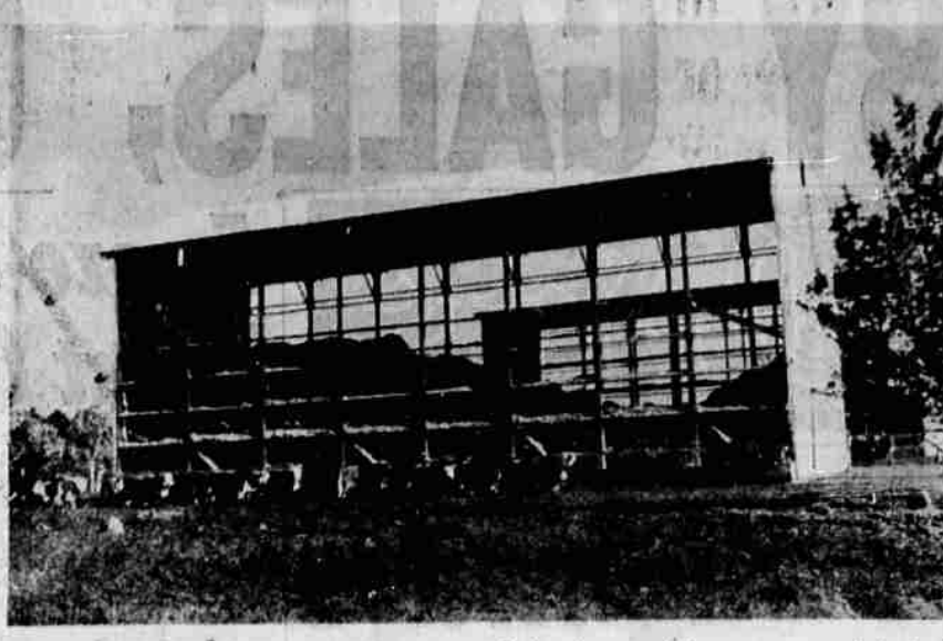
THIS HAY SHED on the Lost River Ranch in Poe Valley has saved its owner a good deal of money by keeping the hay dry during the wet winter, according to County Agent Ray Petersen. The shelter is of pressure treated pole construction, and is equipped with self feeders for chopped hay along the sides. Baled hay can be stored equally well in the shed. Complete plans for a similar building, which could be modified for individual conditions, may be obtained at the County Extension Agent's office in the post office building.
