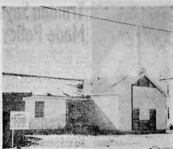
NEW CHAPEL of the Church of Jesus Christ of Latter Day Saints in Alturas will be dedicated in the spring. The building is located at 2001 East Street. Services are conducted by members of the congregation. —Photo by Charles Golden
