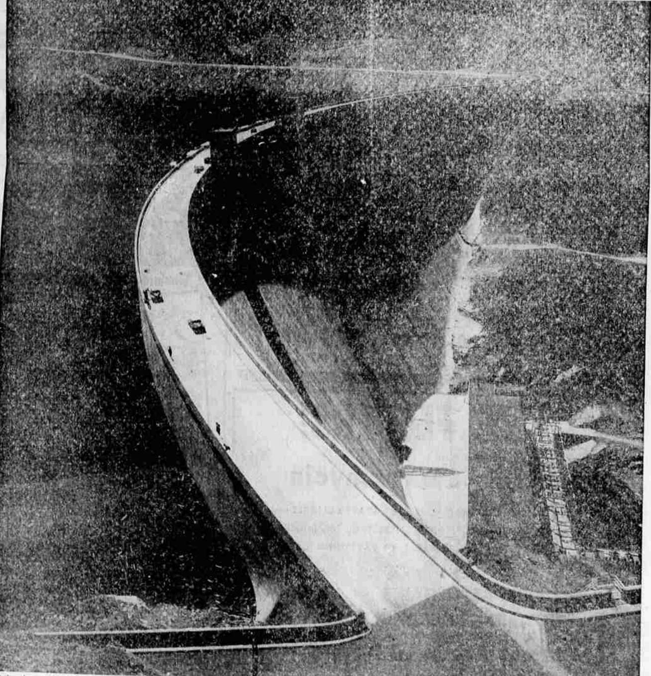
Built and operated by U.S. Bureau of Reclamation, Montana's new Hungry Horse Dam generates over 280,000 kilowatts through its enormous power plant.
