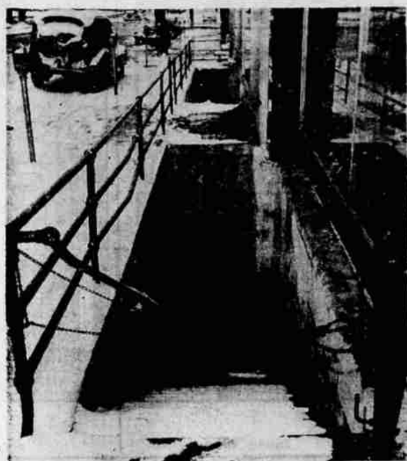
THIS BASEMENT OFFICE located under the present location of Dick Reeder's store at Fifth and Main, was the location of the Evening Herald and The News from 1927 until 1936, when the combined papers were moved to their present location at Main and Esplanade. All editorial, advertising and business offices were in the basement in addition to the pressroom and composing room.
