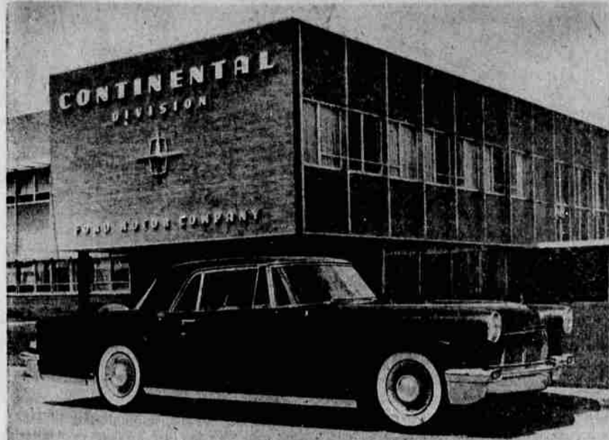
THE CONTINENTAL MARK II, Ford Motor Company's new prestige car introduced last fall, is built in a plant in Dearborn, Michigan, designed exclusively for low-volume high-quality production of this car. Manufactured with special attention to quality, styling and detail, the new Continental retains in modern form the enduring proportions of the former Lincoln-Continental. It is more than 18 feet long and has a hood almost six feet long. The overall height of only 4 feet 8 inches and the width of 6 1/2 feet accentuate its long, low appearance. A unique frame design provides ample room for all occupants. The "modern formal" styling emphasizes the functional use of chrome, steel and glass.
