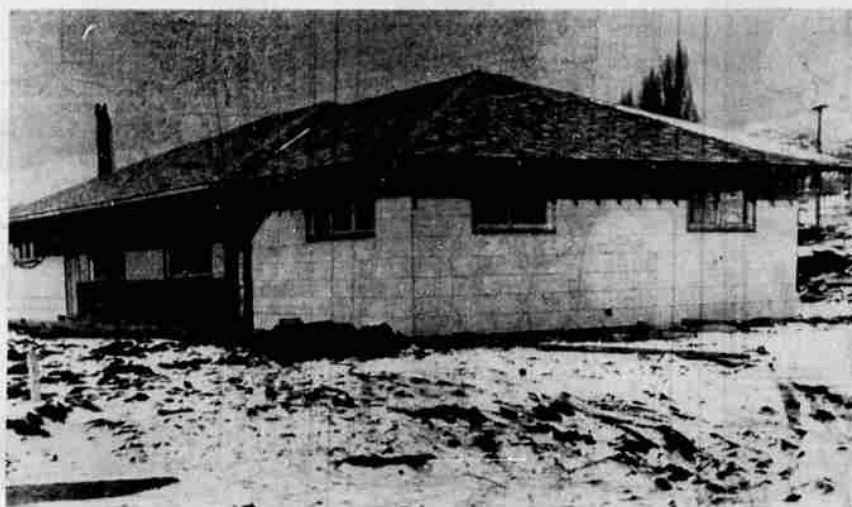
NEW RENTAL HOMES FOR AIR FORCE PERSONNEL , and other new residents coming into Klamath Falls, are being built by John Fowler and Fred Hoagland on Division Street a short distance from Main Street. The first of the duplex units is shown here. The builders plan a group of the new units on this tract. Each unit in the duplexes will have two bedrooms and will be heated from a natural hot water well which has already been dug on the tract, announced d Fowler.
