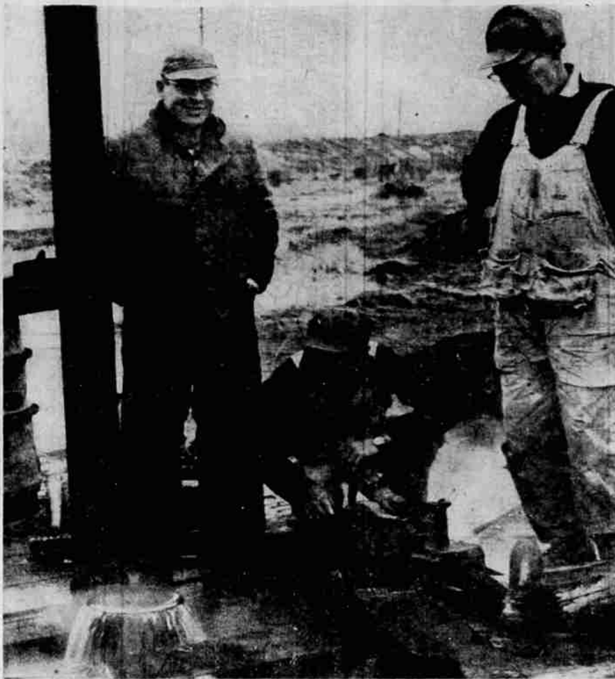
HOT WATER FOR HEATING NEW HOMES was brought in on Division Street by a crew headed by E. E. Storey, Merrill, left. The water, which is flowing to the surface at a temperature of 198 degrees, will be used to heat several duplexes being built by John Fowler and Fred Hoagland at Division and Oak streets. I. C. Wallin and K. J. Rusco look over the artesian well with Storey. The builders are building the duplexes for occupancy by U.S. Air Force personnel and other new residents of Klamath Falls expected to arrive in the city beginning this spring. Each unit in the duplexes will have two bedrooms, announce Fowler.
