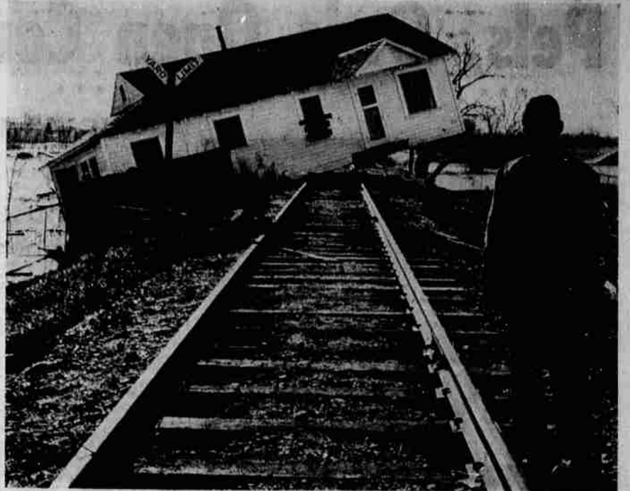
HOME ON THE RAILS was what a Yuba City family went home to after being forced to flee the flood waters of the Feather River in California. Herald and News Photographer Don Ketter took the above picture a few hours after the swirling waters subsided.
