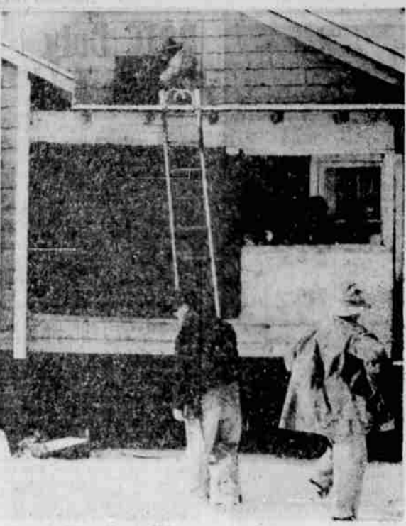
CONSIDERABLE DAMAGE to the front room and kitchen of this dwelling at 2695 Alma Alley was caused by a fire reported at 11:38 a.m. Wednesday.
