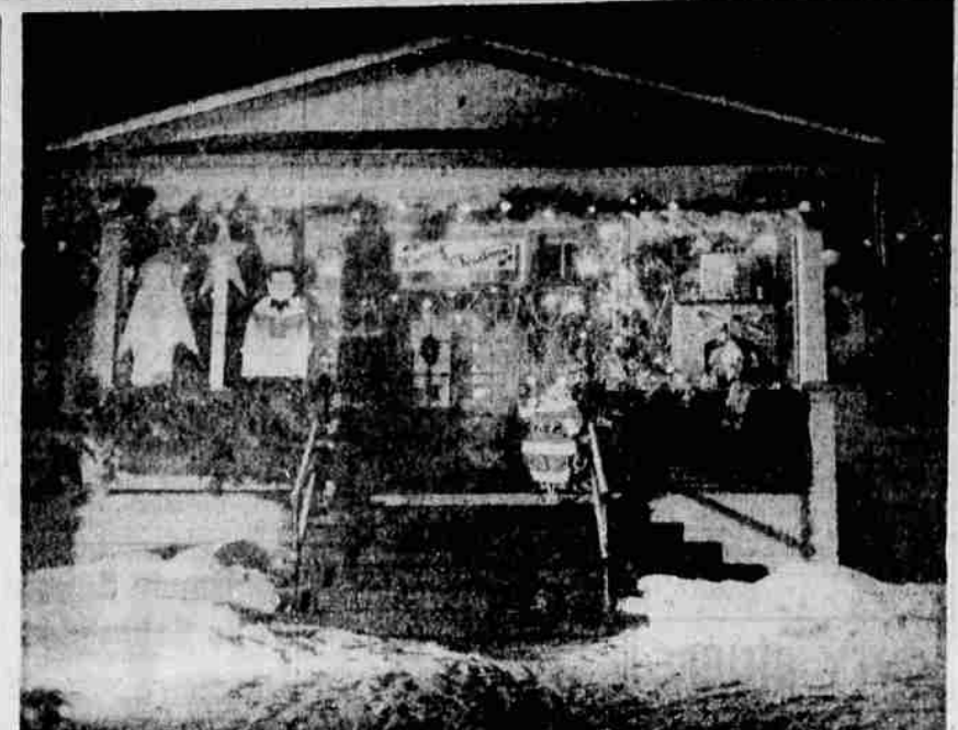
THE SOUTHERN PACIFIC CLUB at Crescent Lake, shown here in its Christmas decorations, was the center of the repair operations last week for crews working on the slide near Cruzette.
