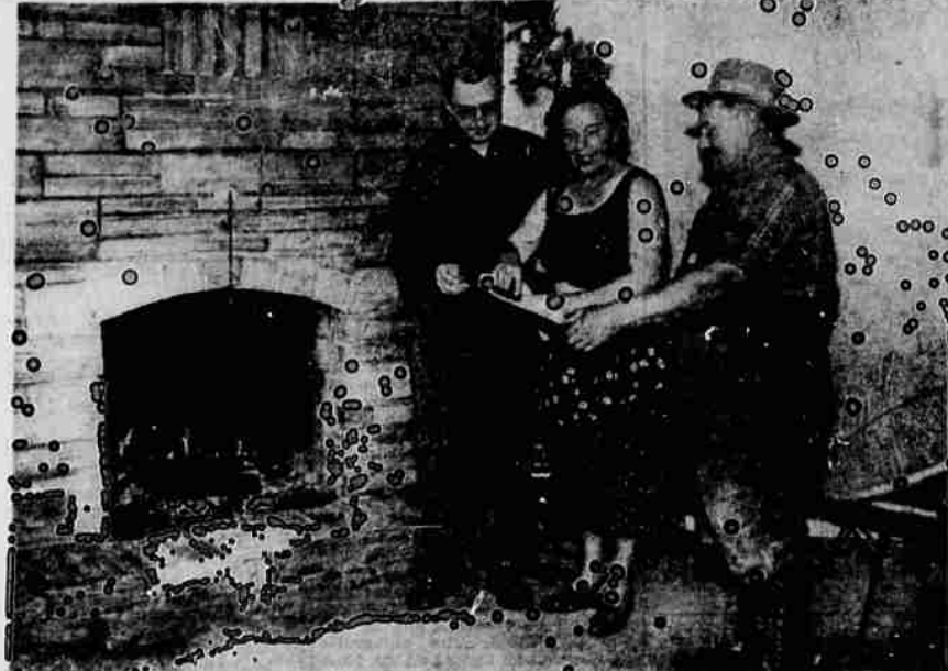
GRACE WELLS, new under construction. It occupies the entire wall of the new room combination, living, dining-sleeping-cooking room. This fireplace reaches to the ceiling and is built to provide heat through three vents. The metal circulator has been used. The opening is lined with brick which will hold heat for hours after the fire dies down. Mrs. Wells, center, looks over plans with Maudie Tipton, left, assistant manager of the Drake Lumber Company and Chas. G. Smith, contractor.
