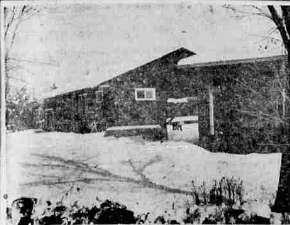
LANDSCAPING on these new homes under construction in the several being built by Mrs. Norma Miller will be completed in the spring by Mrs. W. P. Myers of Lakeshore Gardens. Mrs. Myers has placed most of the trees and shrubs and planted the lawns in this circle of 14 homes.
