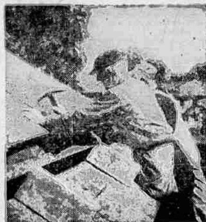
A new roof...
