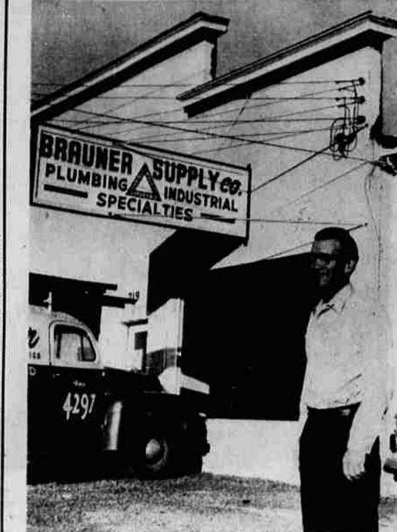
A NEW BUSINESS, Brauner Supply Company, 719 Market Street, was launched in Klamath Falls during the past week. Martin Brauner, owner of the firm, said it will specialize in wholesale distribution of plumbing and industrial supplies. Customers throughout the Klamath Basin will be serviced. Brauner for 18 years was general purchasing agent for a leading Pacific Northwest wholesale hardware company with headquarters in Klamath Falls.
