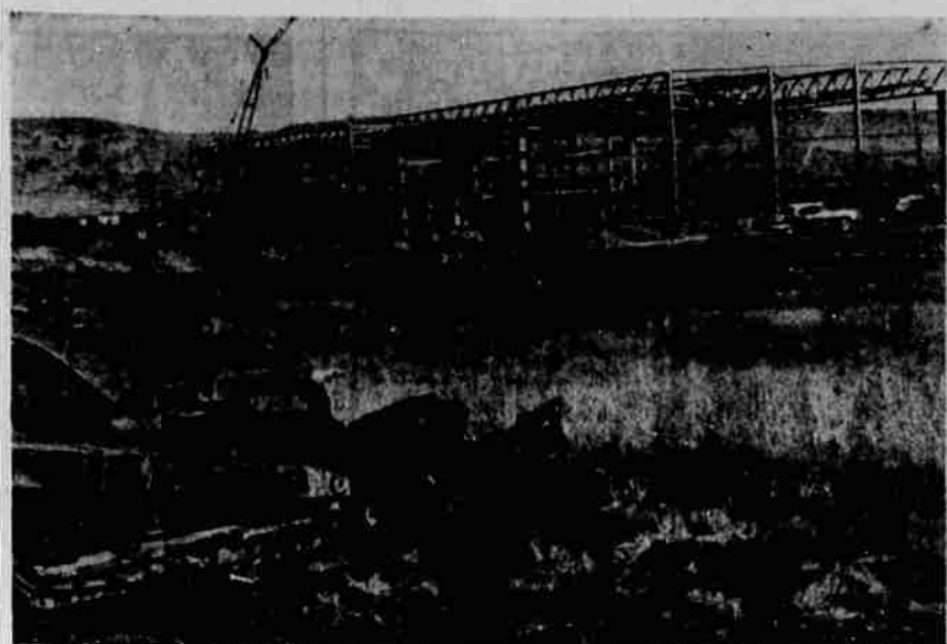
THE FRAMEWORK FOR THE ALERT HANGAR at the Klamath Falls jet intercept base is being built on the north end of the airport. This special heated hangar is the standard type built at all jet intercept bases. It houses two jet interceptor type aircraft in each side, with the quarters for flight and maintenance crews in the middle section. The pilots and ground alert crews will be on duty in the hangar 24 hours a day, seven days a week. The front of the building faces on the alert taxiway, which leads to the main runway. When an alert is sounded the plans designated for flight must be in the air in a maximum of five minutes or the crews must report their reason for delay to the commander, Continental Air Defense Command. The hangar, of steel framework construction, is being built by the Donald Drake Co., Portland. —Photo by Kettler
