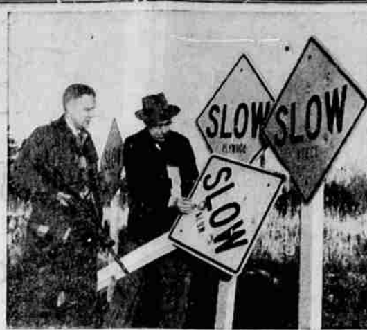
GUNFIRE TEST on highway signs, conducted by laboratory technicians at a northwest rifle range, proved fir plywood's greater resistance to this act of vandalism.
