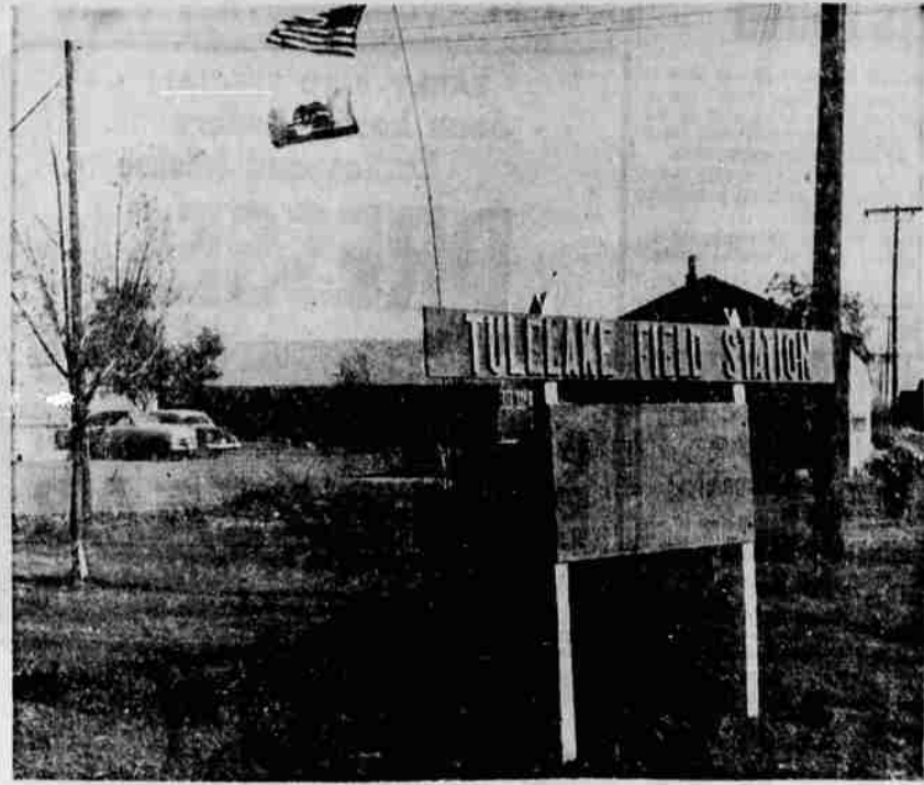
ALMOST READY FOR OCCUPANCY is the new Tulelake Field Experiment Station of the University of California College of Agriculture. The $20,000 addition to the station should be completed by next week, according to Burt Hoyle, manager of the field station.
