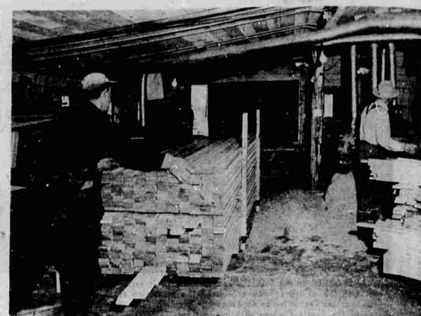
MOULDING FOR BUILDINGS under construction at the airport is being turned out by Chris Moulding plant at 3005 Anderson Avenue. The lumber is being used by the David A. Richardson Company, building contractors at the new jet base. From left (with back to camera) Lloyd Ford, tail-off man on rip saw; feeding rip saw is Richard Florence and at right Chris Litzberger, who with his wife owns and operates the plant.
