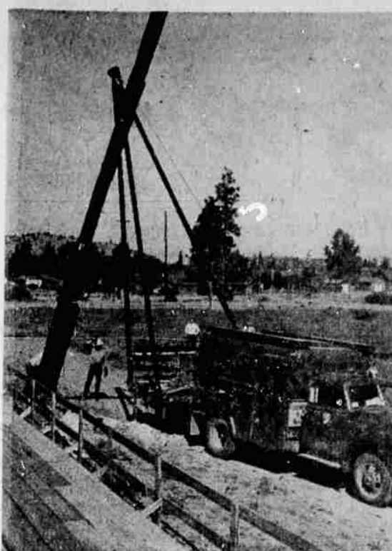
NEW FOOTBALL FIELD LIGHTS have been installed recently at the Weed High School field. California Oregon Power Co. crews strung new lines to the field and erected the poles holding the lights. —Photo by Shasta View studio
