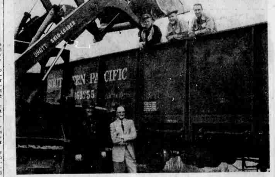
URANIUM was loaded from the White King and Lucky Lass mines near Lakeview this week for shipment to the Vitro Chemical Company at Salt Lake City. Shown at the loading operation of the first three cars of uranium ore to leave Oregon are Pete Vernon of Paisley, tractor operator, and C. Ira Moore, secretary of the Lake County Chamber of Commerce, standing in the S.P. car are, from left, Don Lindsey, Clair Smith and Bob Adams, three of the partners of the Lucky Lass mine which they have leased to Thornburg Bros., Grand Junction. Thornburgs also operate the White King at Lakeview, the two-mine operation combined under the name of Lakeview Mining Company. —Photo by Buell
