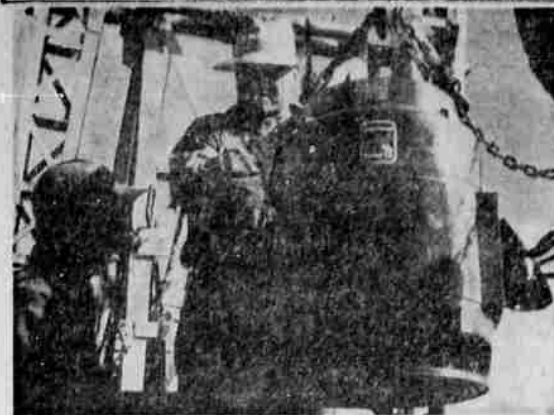
TRUMAN KIMSEY, left, of Silver Lake, and Richard Schaub, of Fort Rock are shown lowering a 30-horse power electric motor for direct connection with a turbine pump at Schaub's new irrigation well. Designed for 1450-gpm with a 74-foot lift, it is the first large electrically driven pump to be installed in north Lake County. J. C. Amaral, general sales manager of Western Pump Company, assisted with the installations. —Photo by Parks
