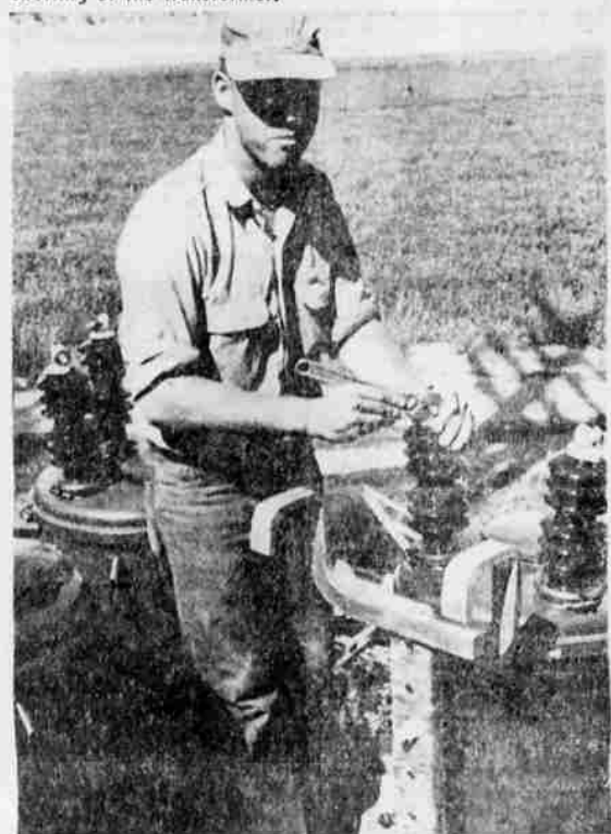
WORKING on the transformer installing crew on the REA-financed power line construction in the Silver Lake area is Daniel Williams, 2105 Hope Street, Klamath Falls. He will enroll for his second year at OTI at the beginning of the fall term. His course is radio and television. —Photo by Helen Parks
