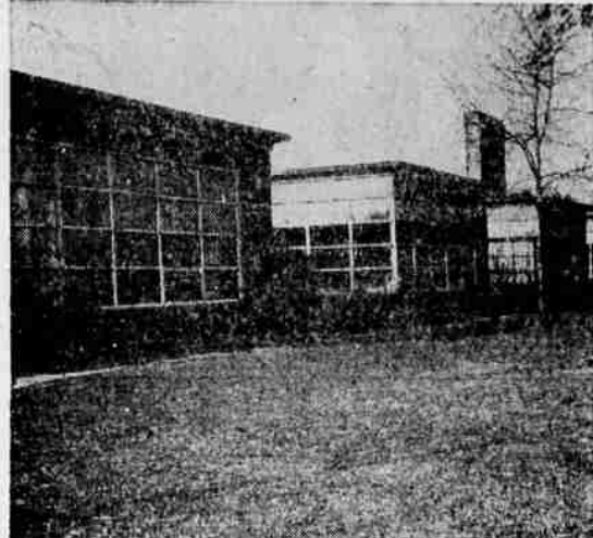
CAMPUS PLAN OF THIS Illinois school provides outside doors for each classroom so that dismissal and play periods don't cause congestion in halls. Building for Crow Island elementary school looks much like small homes, giving a warm atmosphere.
