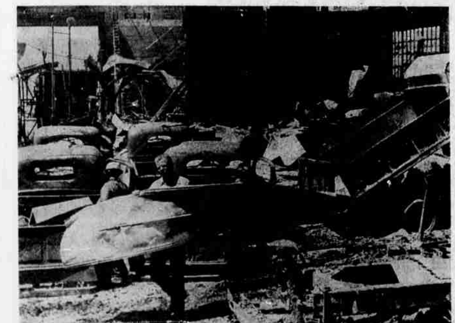
NOTHING BUT CHARRED WRECKAGE was left after the fire that razed the repair shed at Tulana Farms Sunday night. This picture, taken Monday morning, shows some of the various equipment that was destroyed in the big blaze. Stuart Hensel is shown packing out a piece of the wreckage.
