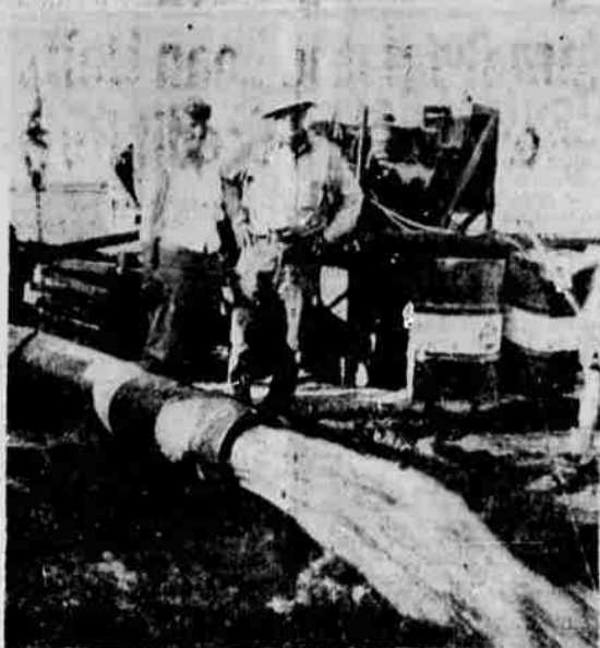
A NEW WELL on the property of Earl LaBranch, Westside rancher near Lakeview, is producing a flow of 3,600 gallons per minute. The well was drilled by Walter Wilson of Merrill. Test pumping equipment was supplied by the Interstate Pump Company of Klamath Falls. The well is 463 feet deep and is cased with a 12-inch casing. LaBranch and his daughter, Earline, are shown at the testing site. —Photo by Buell
