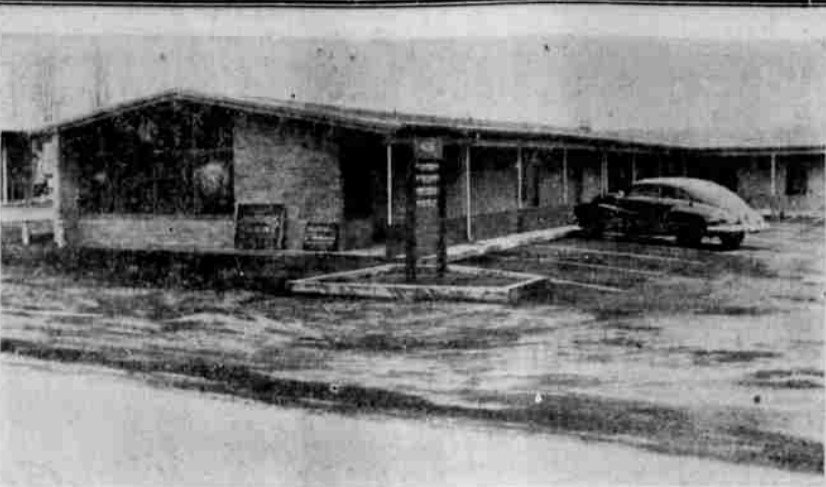
THIS CALIFORNIA STYLE building at 4036 South Sixth Street will be future offices of seven Klamath Falls doctors. The building has a wide, surfaced parking area for accommodation of 40-50 cars. Construction conforms to other buildings in the new development of South Sixth. Offices will be ready for occupancy in the next few weeks. The property is owned by Dr. G. O. Erlandson.
