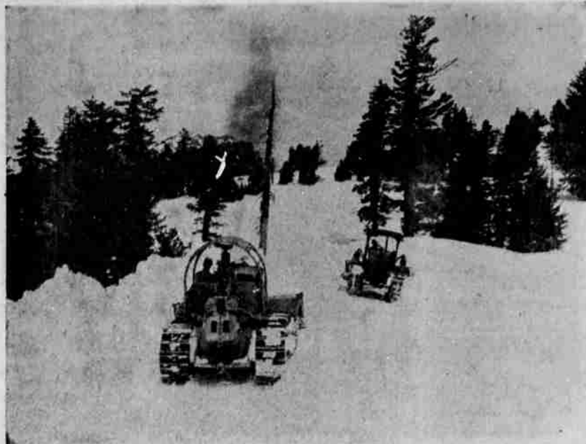
THESE MEN WORK IN A FIELD OF WHITE as they break the first trail over twelve foot deep snow up at Crater Lake. The bulldozers make a trail and then push the snow back into the rotary plow that follows them up.
