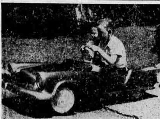
SPORTS car of styrene and fiberglass is propelled by bicycle drive that is adjustable to child's size. It's six and a half feet long, weighs 65 lbs. and comes in red, yellow or blue, all gold trimmed. Materials are same as today's adult dream cars.
