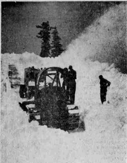
WHILE A BULLDOZER PUSHES snow in one direction a rotary moves in from the other to toss the snow high out over the bank. This scene was snapped during the opening of the North Entrance at Crater Lake last spring.
