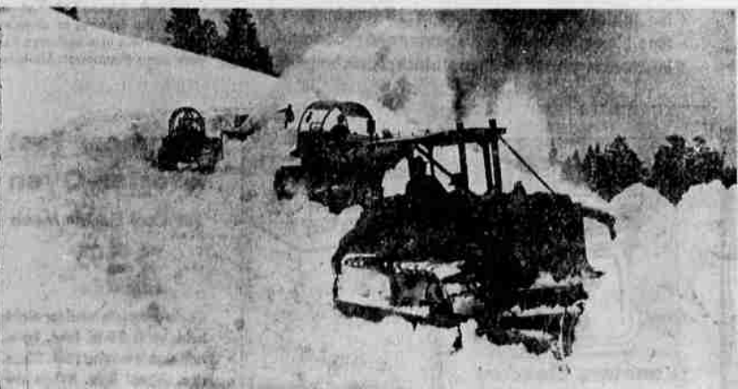
THREE BULLDOZERS AND A ROTARY were at work on this stretch of the rim road when the time came to clear off the winter's accumulation of snow.
