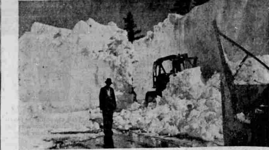
MACHINES AND MANPOWER are the prime requisites for keeping open our highways when the snow starts. This crew is busy hacking out a junction somewhere in the high hills.
