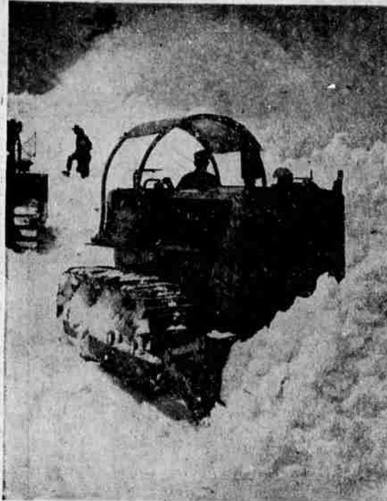
WITHOUT THE RUGGED "CATS" it would be a terrible chore to keep the roads open in the winter months around our High Desert. This blade-equipped cat, however, will move a lot of the white stuff in the course of a day.
