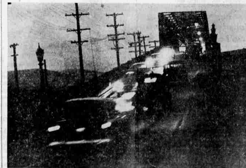
STARK OUTLINES AGAINST A NIGHT SKY, the dark forms of telephone poles and steel framework of crowded South Sixth Street viaduct form a sharp contrast to the blur of automobile lights. The shot was taken looking towards Klamath Falls with a 4x5 speed graphic camera at 1/2 second at f5.6.
