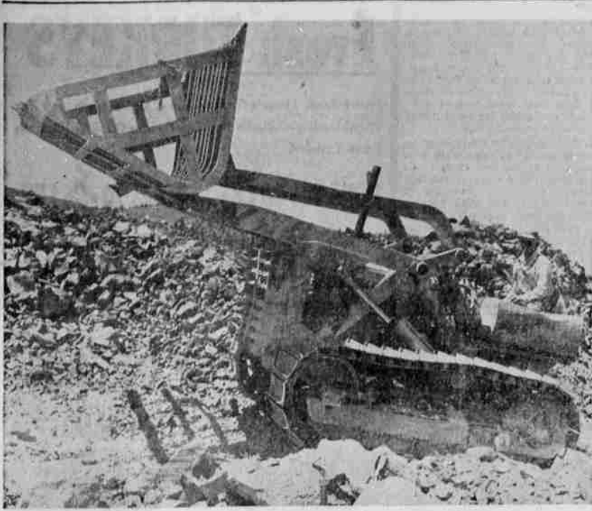
THIS HUGE, OPEN STEEL basket operated by a Caterpillar tractor scoops up chunks of scoria and dumps them into trucks for the haul down Glass Mountain. The abrasive material is cut into bricks at the Newell plant of the United States Pumice Supply Co., to be shipped to many parts of the world for cleaning cooking grills.
