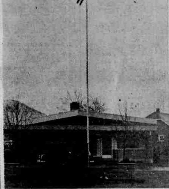
THE AMERICAN FLAG flew on Veterans Day for the first time from the new 42-foot steel flagpole which has been set in a concrete base in the veterans' section of Klamath Memorial Park.
