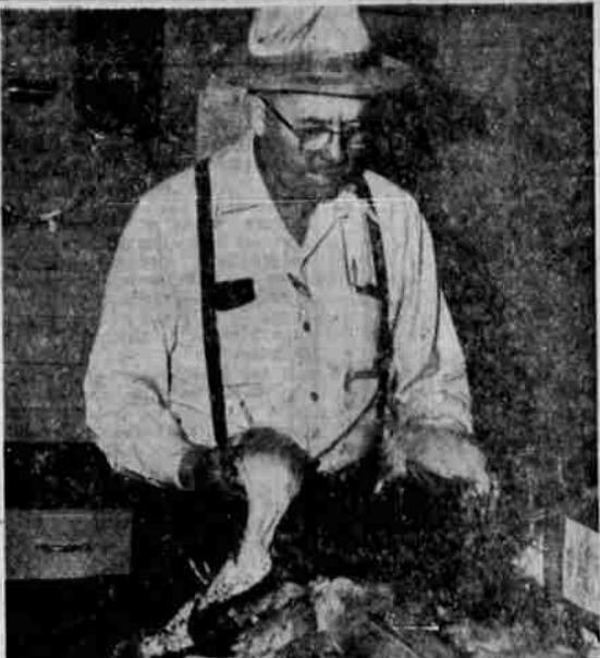
JACK CIER — manager of the Legion Club looks over some mallards and pintails, just picked clean by a mechanical picker operated by Mrs. Cier. The business, in a specially constructed building in the rear of the Bank of America is swamped with birds during the migratory waterfowl hunting season.
