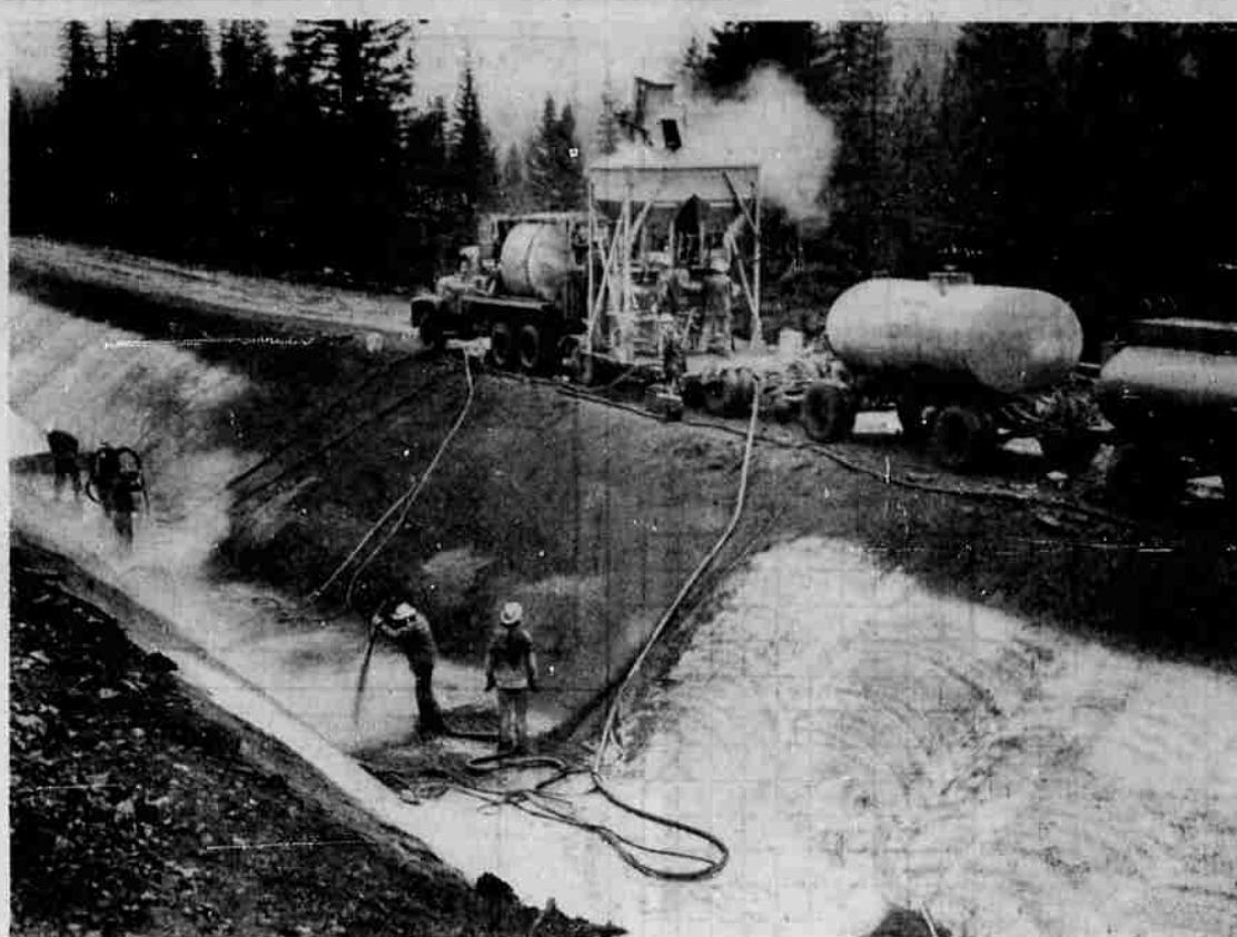
A STRONG MAN'S WORK this business of spraying Gunite on the walls of the canals at Copco's Lemola project. This picture shows the crew spraying the concrete and water mixture over the steel braces laid along the ditch walls. This picture was taken below the Lemola Dam on the canal leading toward Lemola number two.
