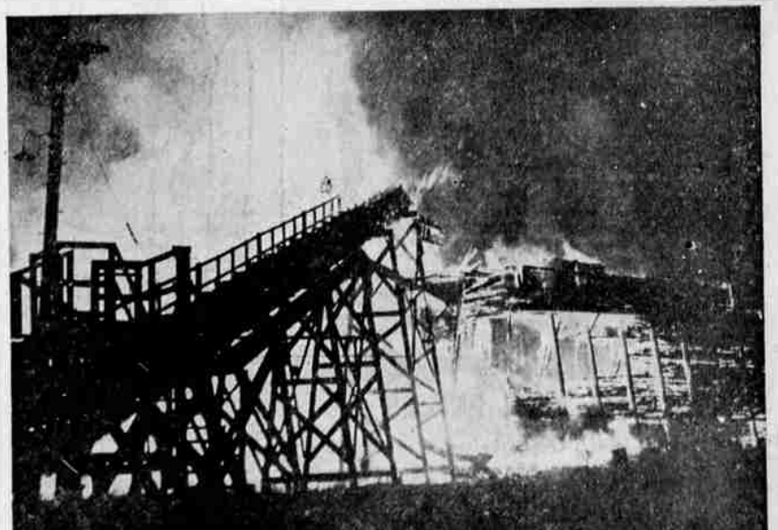
THIS OLD FUEL BIN on the Modoc Lumber Company property on Lake Ewauna went up in flames last night. The bin was on the old Ewauna Box Company, Hercules Powder Company mill sites and is now owned by the Modoc Lumber Company.
