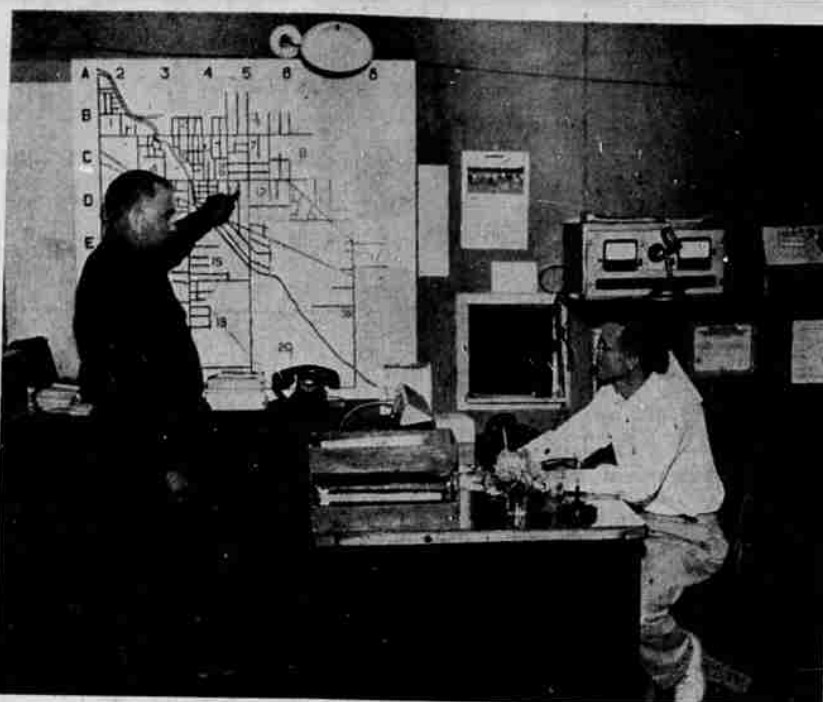
LEO KAMARAD, rear, shows Fire Chief "Buster" Gordon how wall chart is marked to correspond with a niched wheel that flips the fire siren to call volunteers to scene of a blaze.
