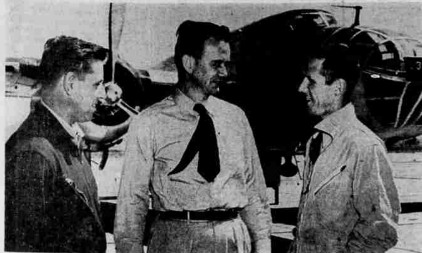
FROM HAMILTON FIELD Tuesday to inspect the concrete hangar at the airport were, from left, Captain Charles B. Nichols, Major R. W. Stewart and Major William Lacey. The Air Force will take over the concrete hangar with reactivation of the airport as a jet interceptor base. Hamilton Field officers expressed approval of the hangar facilities on their brief visit to Klamath Falls.
