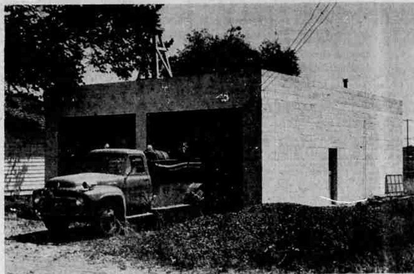
A STOUT BUILDING of pumice brick now houses the Bonanza Fire Department's equipment. There is still a good deal of gear to be added, but the volunteer unit is rapidly filling its needs and can give excellent protection for their area.
