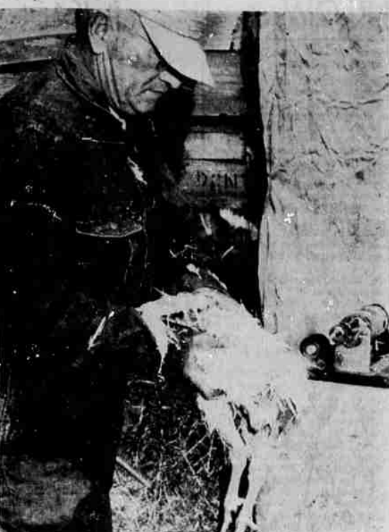
THE FEATHERS FLY as Scott W. McKendree demonstrates his latest production, a home-use chicken picker. McKendree, who already has a duck picker on the market, put in over a year's research on the chicken picker before turning out these pilot models. The picker, designed for average home use, should be in production on a commercial basis within three months, he said. The picker works from any low powered motor, such as a home drill, and takes off pin feathers by use of a four bladed rubber stripping wheel.
