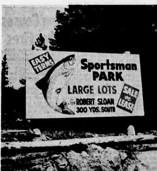
A NEW DEVELOPMENT is planned for the Westside area with the start of Sportsman Park, a summer home site project. Bob Sloan, the owner and operator, will have 24 lots up for sale this year, with more to be added in the future. The park will feature a shade and grass strip along the highway at the Rocky Point Junction, with home sites ranging up the hill and back toward Cold Spring.
