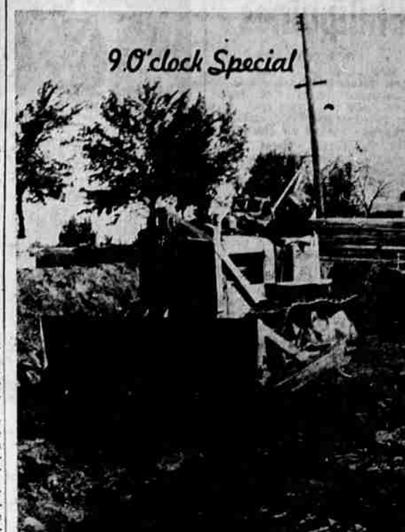
9.0'clock Special GRADING THE SITE of a new house for Carl Long at Tunnel and Prospect Streets was Fred Seutter, bulldozer operator for Graham Brothers.
