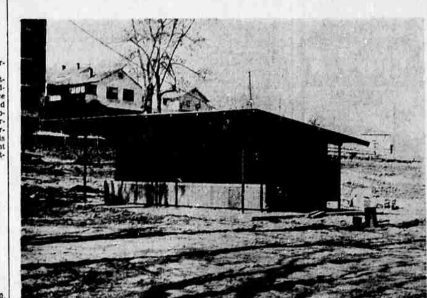
DUE TO OPEN SOON is the combination kitchen and rest rooms building at Veterans Memorial Park, located on Main Street by the Link River bridge. The low, modern construction has walls of Roman brick and cement floors. The kitchen has four cooking units and will have two double compartment sinks. There are two rest rooms. Plans for the building were drawn by Vern Schortgen, city building inspector.
