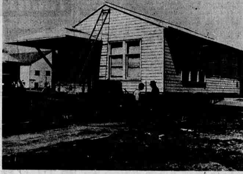
ON THE NEW SITE and ready to go is the Klamath Sportsmen's new clubhouse and headquarters, recently moved to the lot above Frei's store. Extensive remodeling is planned for the surplus structure, and it is hoped it will be ready for use by mid-summer.
